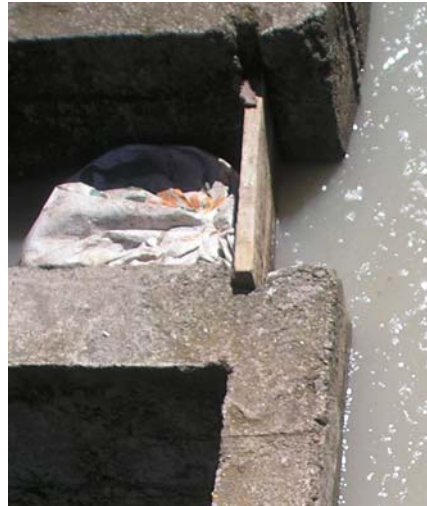
Figure 11 Wooden + Sand Bag Flow Gate
