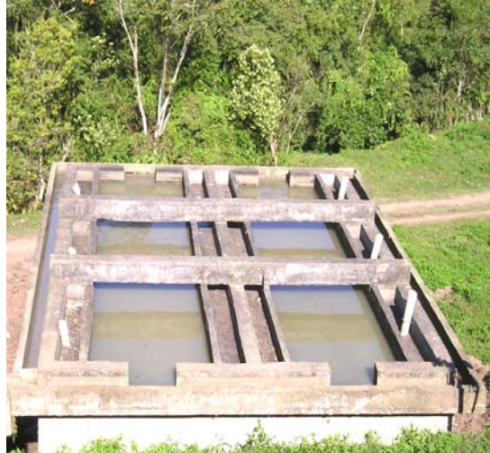
Figure 5 Photograph of Parallel Imhoff Tanks, Las Vegas
